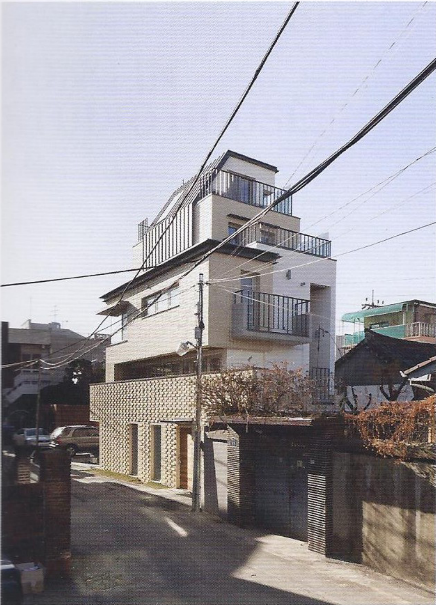
The building gradually reduces floor area from the third to the fifth levels by installing terraces.
